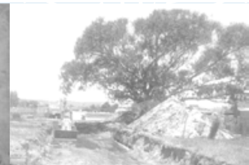
Drainage work on the College oval in 1977.
