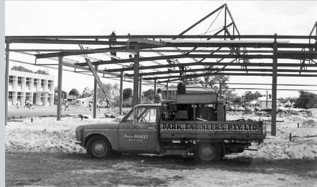
The Connell Centre under construction in 1977.
