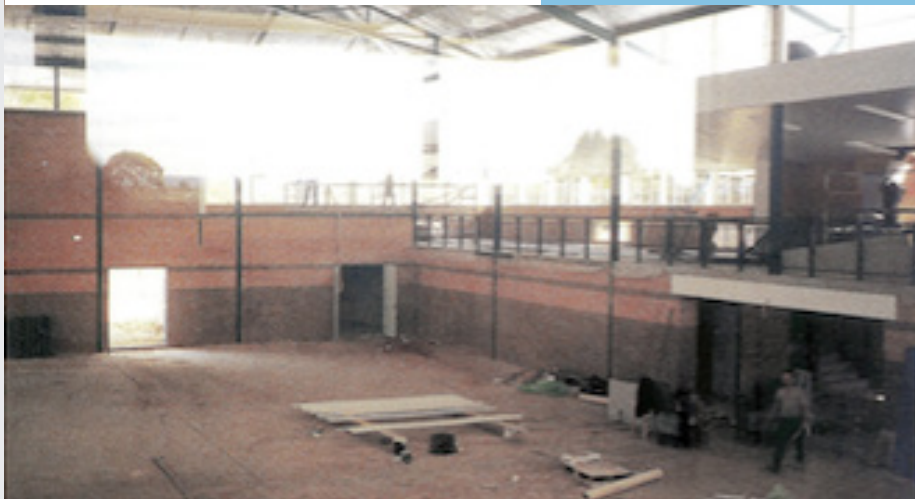
The Fr Peter O'Reilly Centre under construction.
