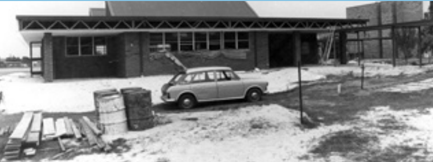
The Prémontré Library under construction in 1982.
